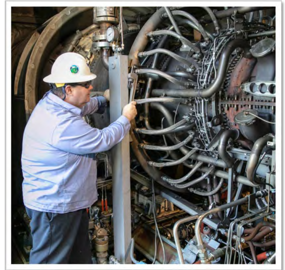
Maintenance work at Cane Island Power Park.
