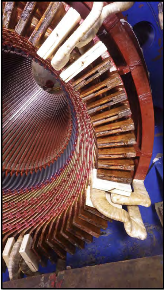
Top to bottom bar axial misalignment on the connection end.
