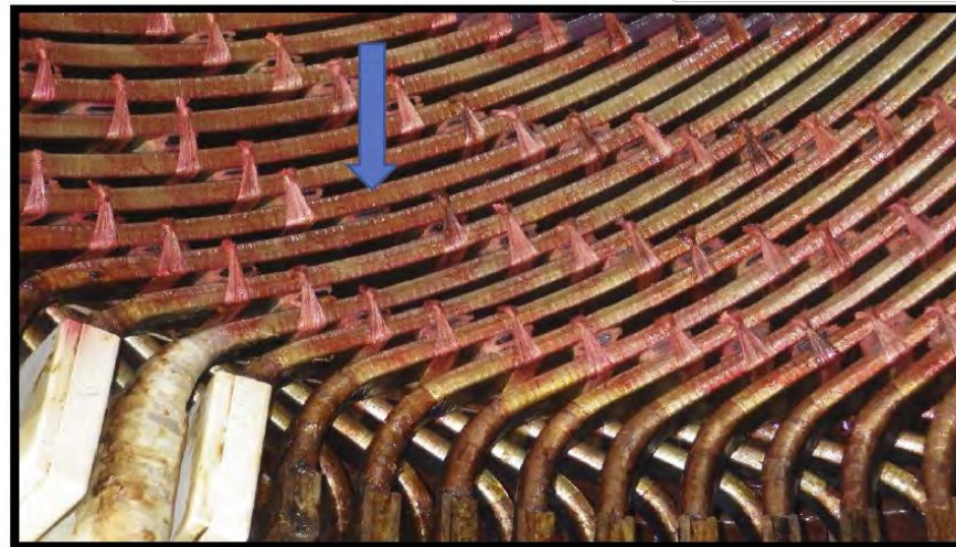
Tie missing after bake
