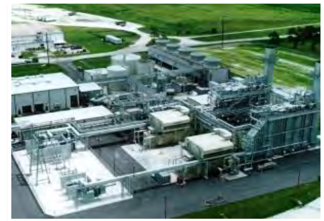
Orange Cogeneration Facility
