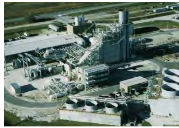
Mulberry Cogeneration Facility
