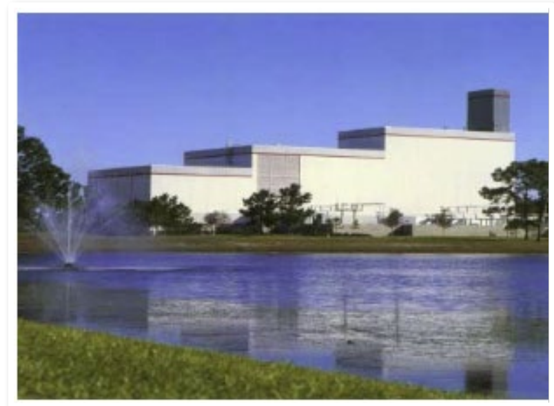
Orlando Cogeneration Facility
