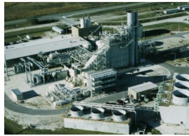
Mulberry Cogeneration Facility
