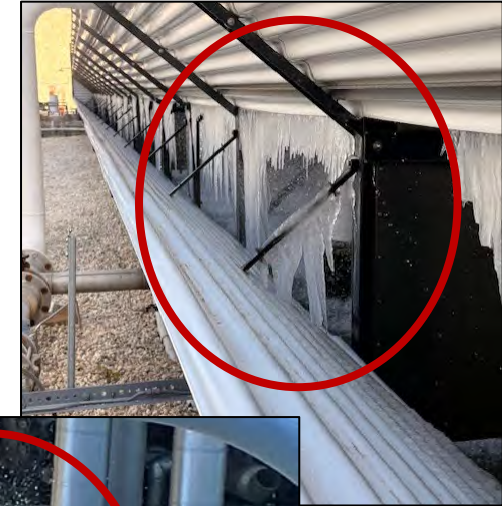
Cane Island 4 - various instrument tubing failures
