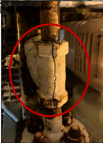
Iron piping froze and cracked
