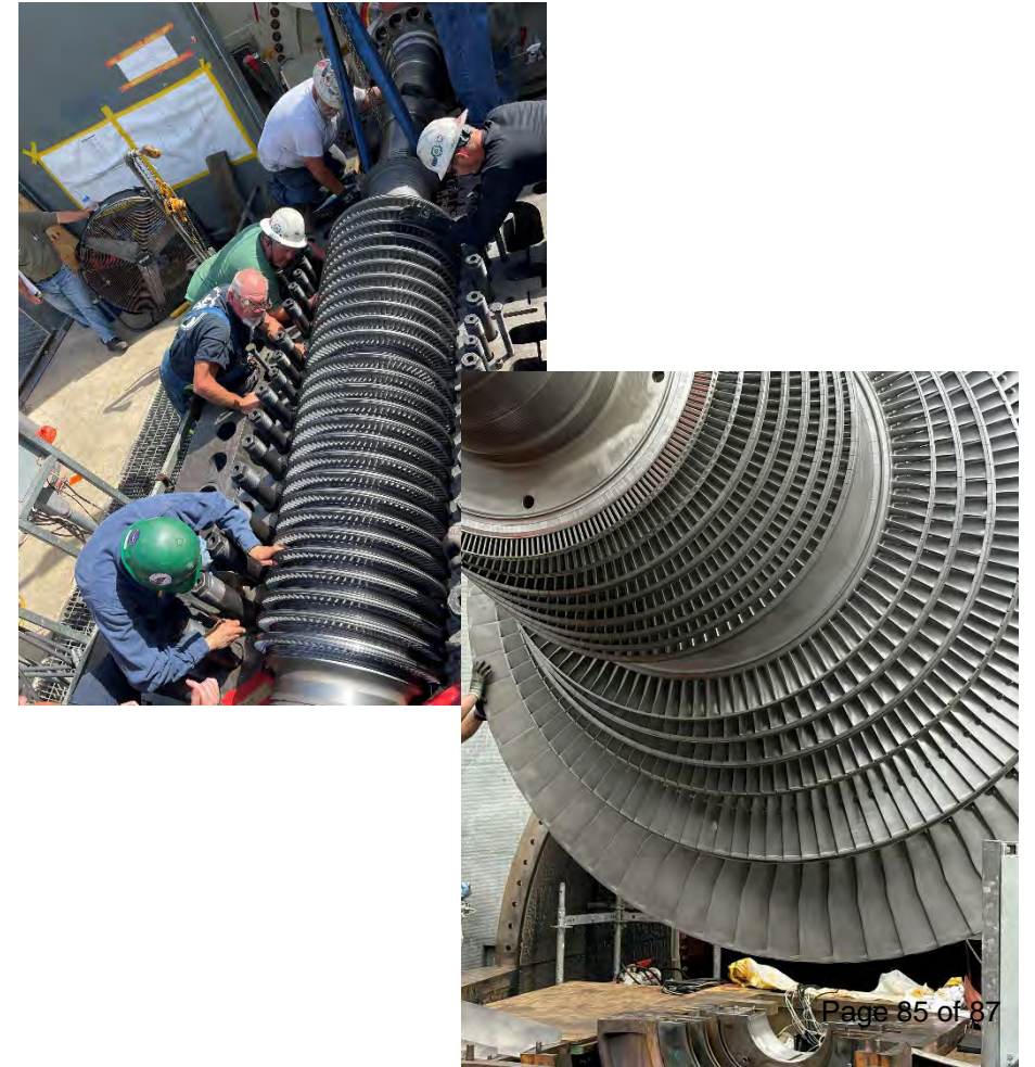
Replace Blades on Both HP and IP/LP
