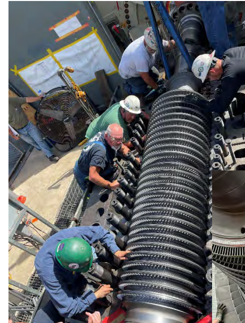
Replace Blades on Both HP and IP/LP
