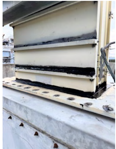
T2 - Top of Low side Leaking fix
