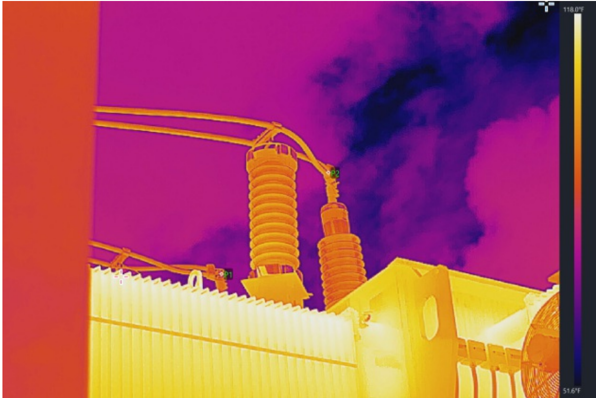
T2 - GSU - HIGH SIDE BUSHINGS
