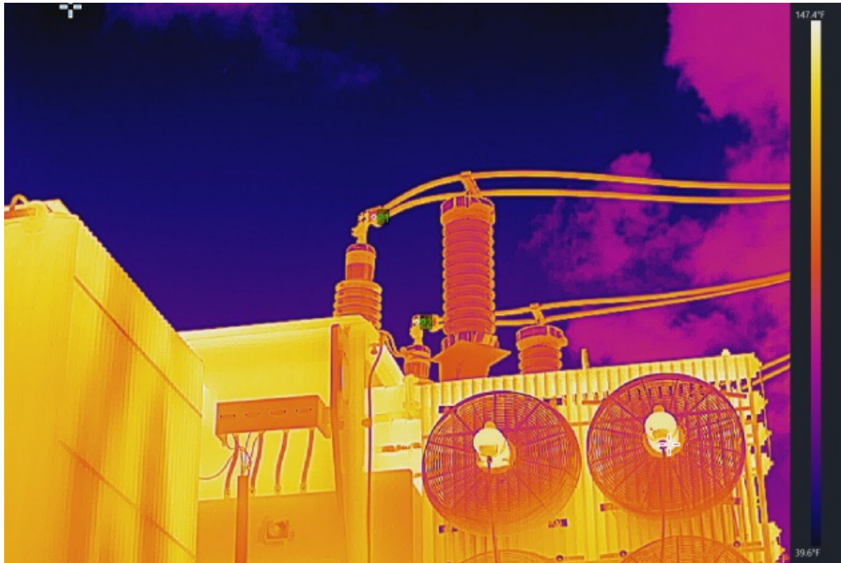
T2-GSU - HIGH SIDE BUSHINGS
