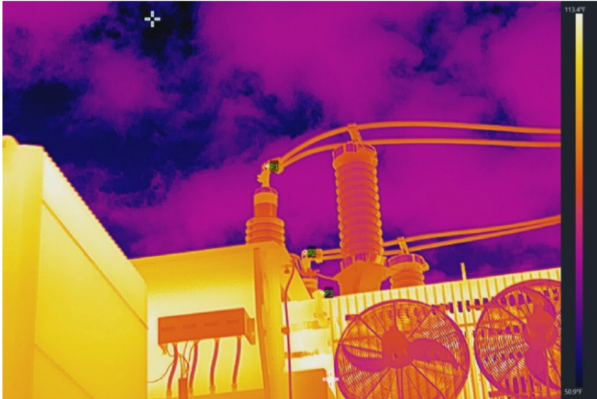
T2 - GSU - HIGH SIDE BUSHINGS
