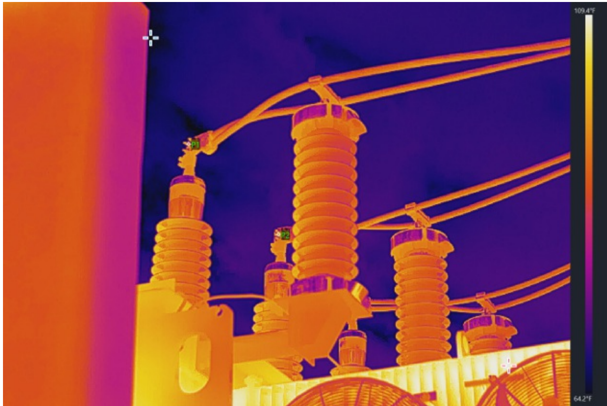
T1 - GSU - HIGH SIDE BUSHINGS
