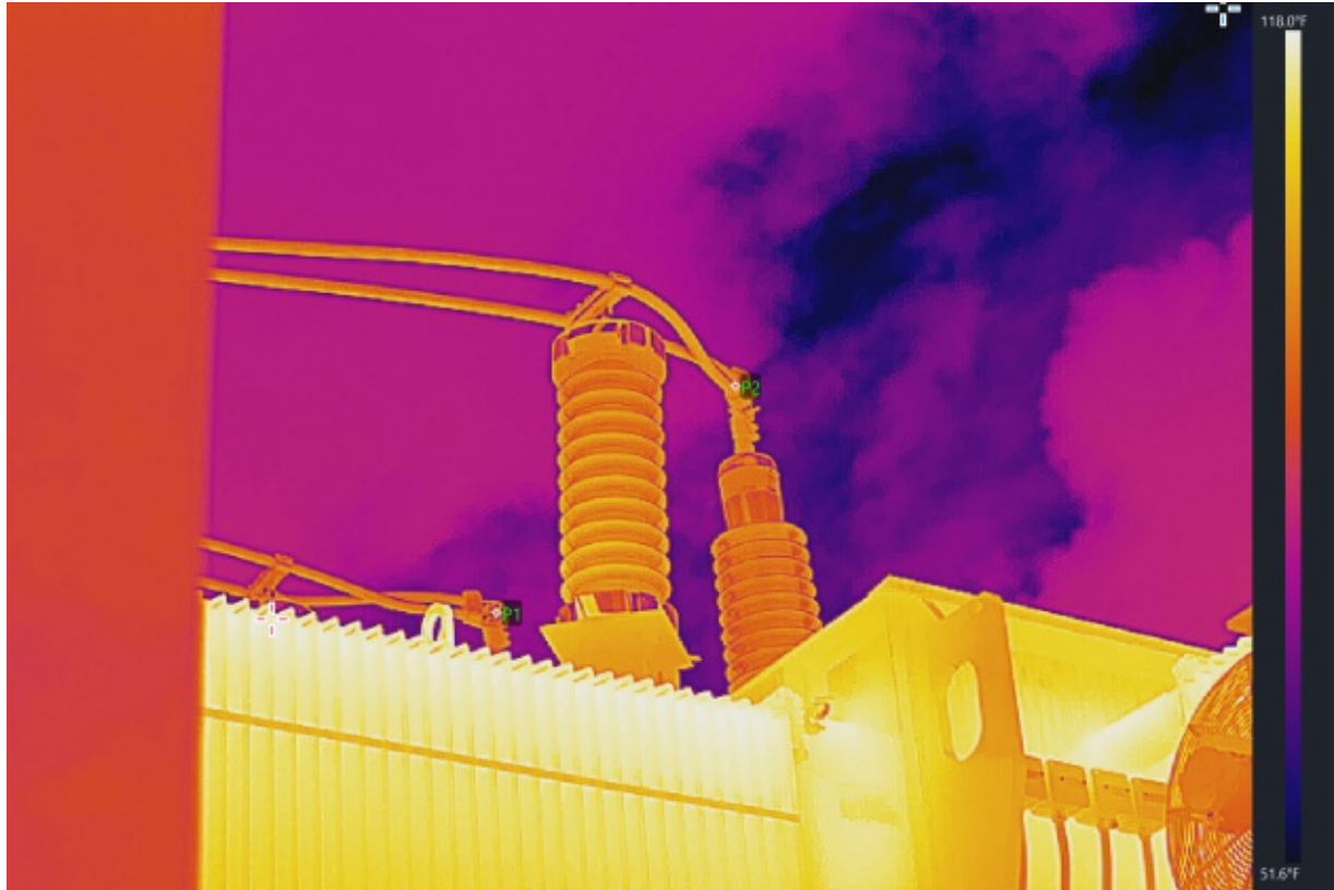
T2 - GSU - HIGH SIDE BUSHINGS
