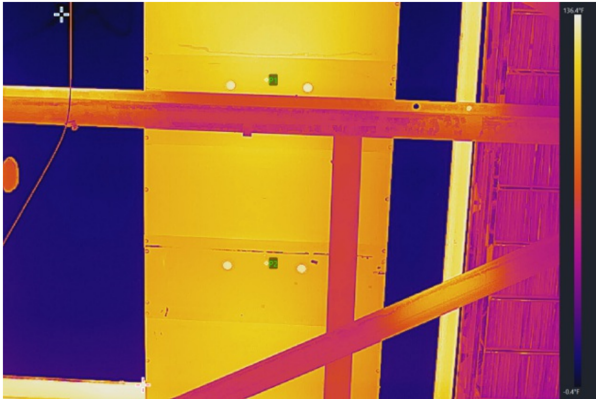
BUS DUCT HEATERS
