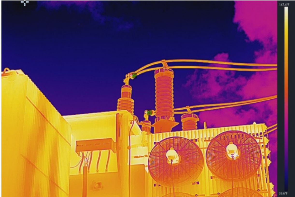
T2-GSU - HIGH SIDE BUSHINGS
