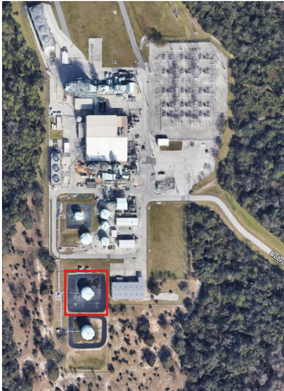
Figure 1: Tank Location in the Plant
