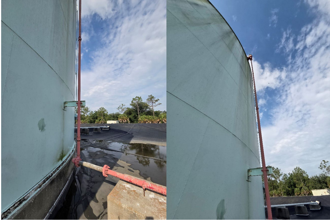
Figure 4: Fire Protection to Be Removed
