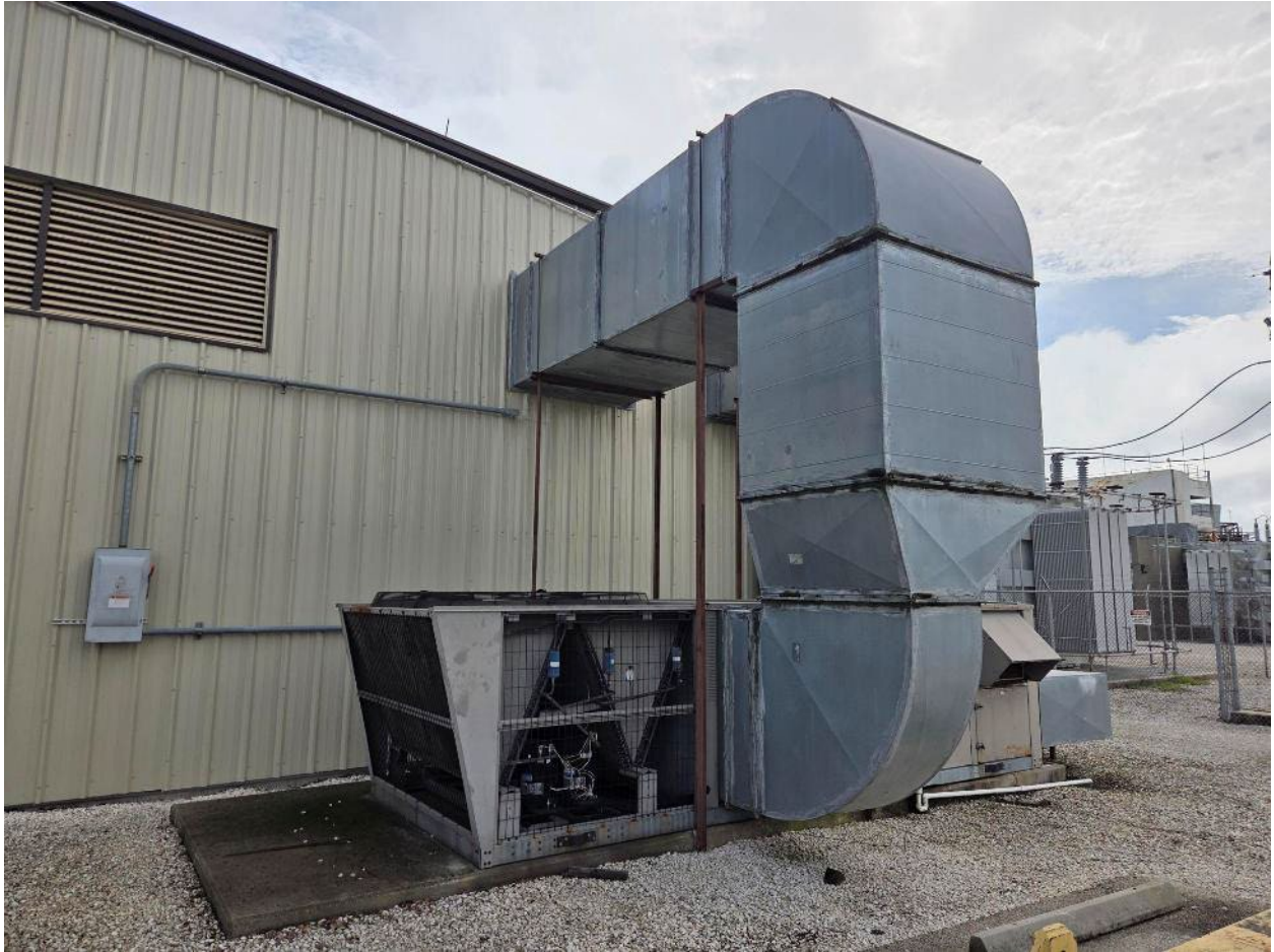
Figure 2: Existing Unit and Ductwork
